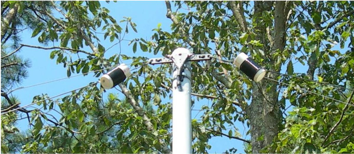
The kit is held onto the PVC conduit using two stainless hose clamps and I topped off the conduit with a white PVC 2 inch cap to keep rain from entering.
